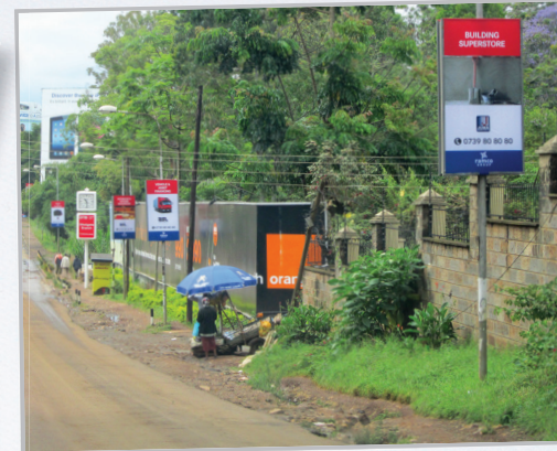
The new Ramco Group street lights outside Westgate shopping mall
